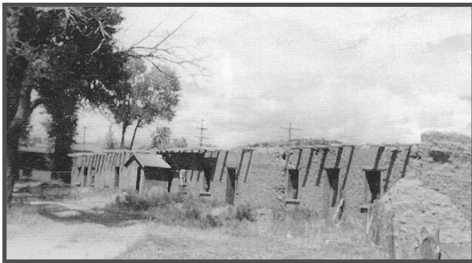
Telephone poles behind the west wall of the cavalry barracks stand as mute reminders that Fort Garland had entered a new and neglectful period but the end of the 1920s saw the birth of a museum.
