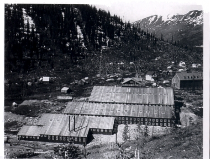
The newly built Gold Prince Mill in 1904 with the Gold Prince Boarding House on the right. ~Photo courtesy of San Juan County Historical Society
