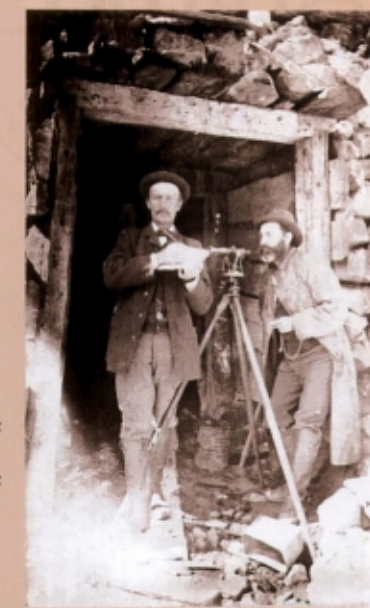
Colburn Allison (left) and Winfield S. Patterson survey the portal to what is believed to be the Columbus Mine. The two men owned a number of mines in the area including the Columbus Mine and Mill in Animas Forks. ~Photo courtesy of San Juan County Historical Society
