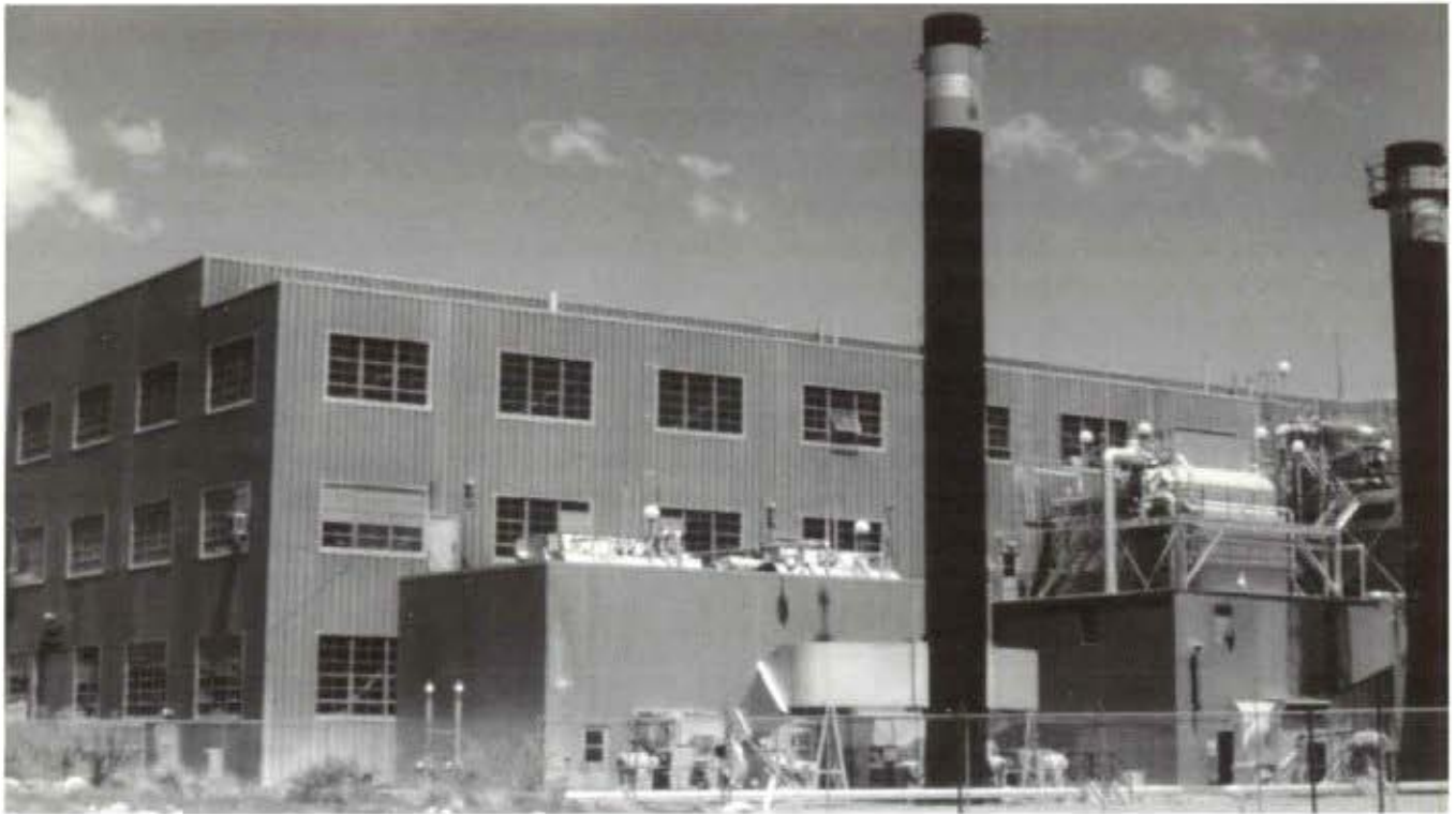
The Basin's first steam plant located in Farmington. Built in 1957, its 32 megawatt output would be exceeded within eight years. Fired by natural gas, this plant remains in operation today.
