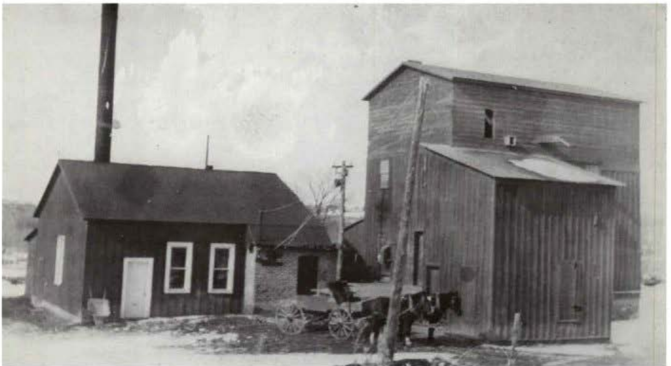
Aztec Light and Power Company's generating plant on South Lightplant Road around 1916. The building on the right is the Aztec Roller Mill.
