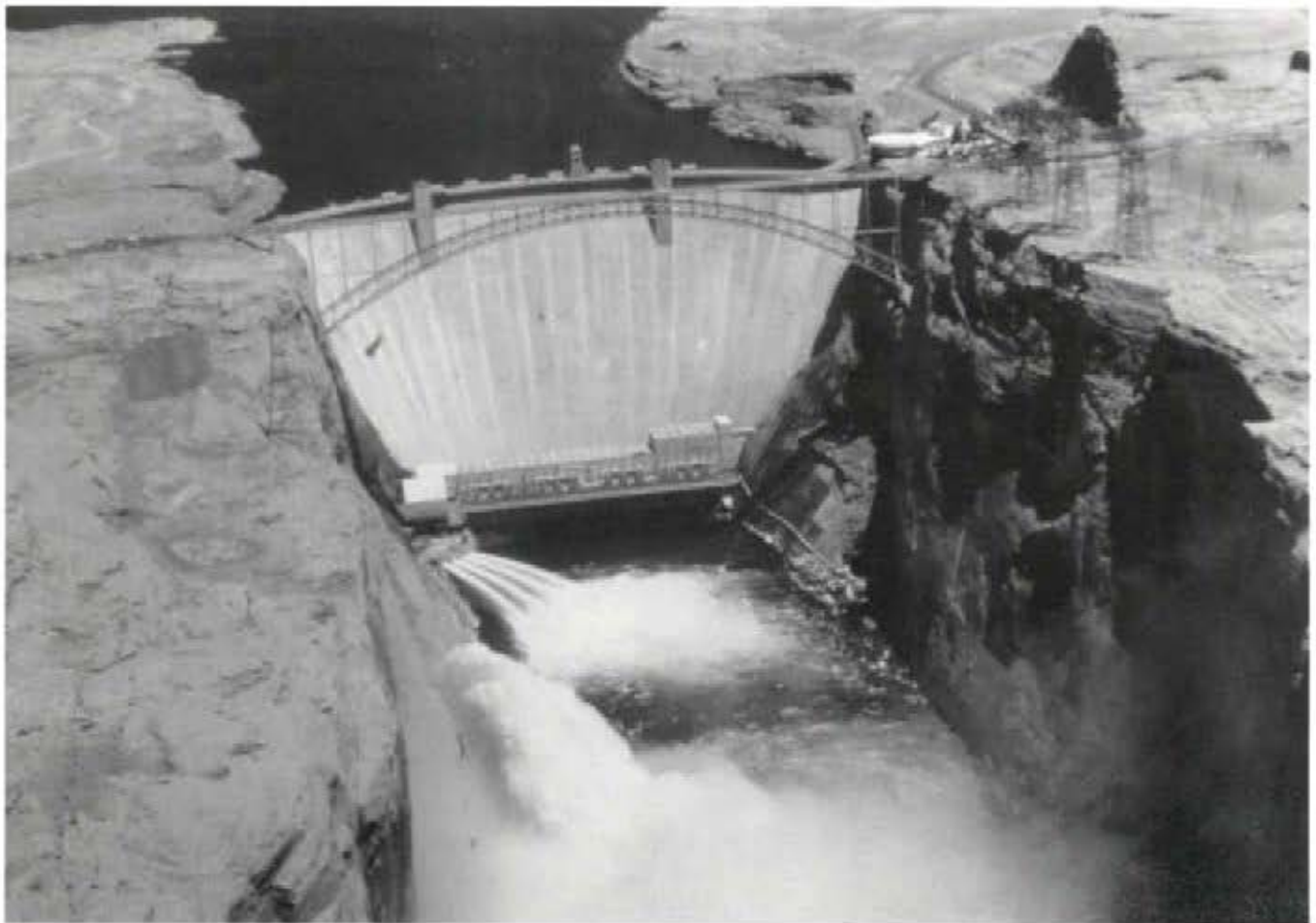
Glenn Canyon Dam on the Colorado River was constructed in the mid 60's and is a major source of W.A.P.A. hydro-power. This is a test flow at 50,000 cubic feet per second in 1984.
