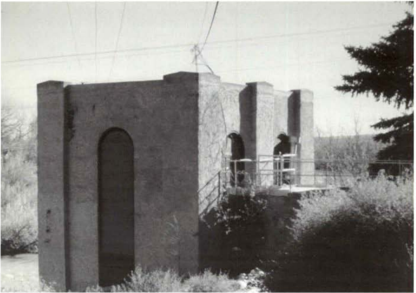
Exterior view of the Farmington Hydro Plant just north of the steam plant. This unit was overhauled in the 80's and still produces its original 300 kilowatts. A giant in its day – now dwarfed by the Basin's nearly 90 megawatt demand.
