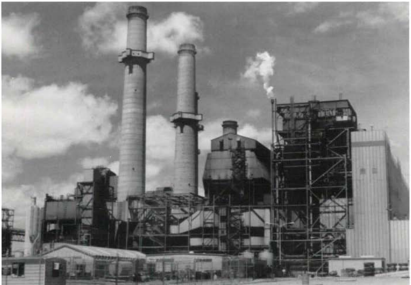
Public Service Company of New Mexico – San Juan Generating Plant, near Fruitland, built in 1972, would add around 1,600 megawatts to the Basin's capacity.
